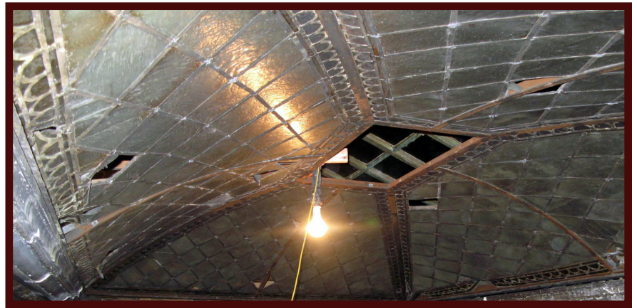
The skylight in its pre-restoration state.
