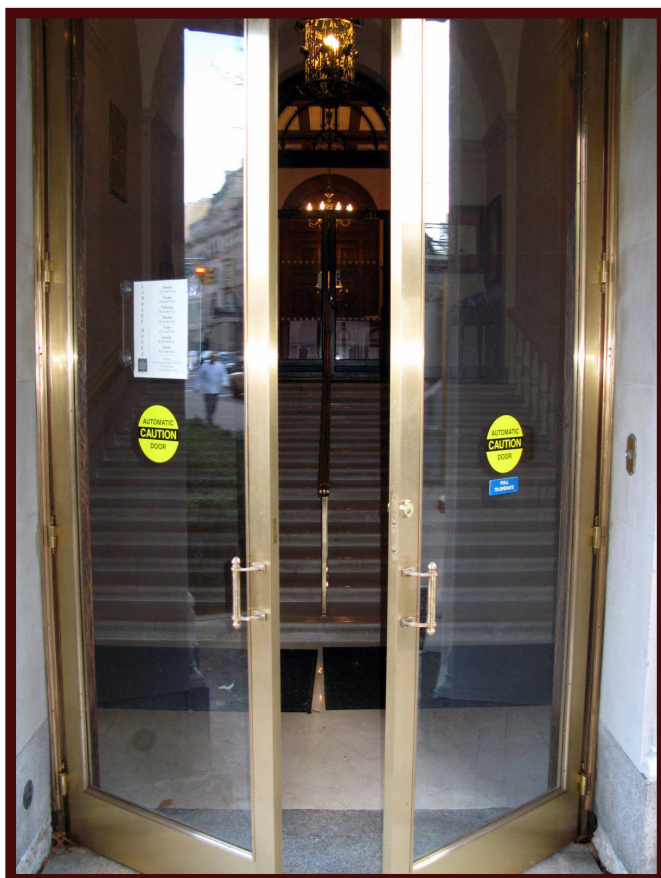
They are taking some getting used to, but these automated doors are a crucial part of making the Library handicap accessible.
