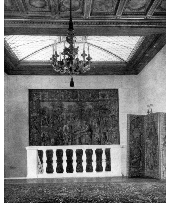
This summer's renovation will restore the amber-colored skylight over the main stairwell. This image dates from when the building was the private home of John S. Rogers and his family. The photographer was standing beside what are now the doors to the Members' Room.
